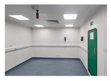
Project scope included remodelling four small rooms into two larger rooms; the combined room was designed to be Grade C with all finishes to match the existing GMP areas. As part of the project, new services were introduced in various key locations to serve new and relocated equipment use as part of the process stream.
