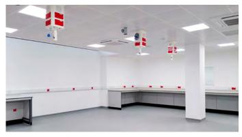
The ventilation system involves connecting into the existing building system providing fume cupboard extraction and tempered supply fresh air to the laboratories, with ceiling-mounted cassettes and corresponding external condensers, to provide duty standby cooling mode of operation.
