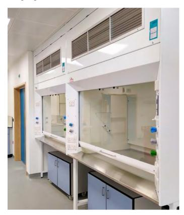
Utilities include a dedicated power supply from a generator-backed supply, water services, laboratory gases, including nitrogen, compressed air, and vacuum which were all piped from the existing infrastructure within the R&D building. A new  $\mathrm{CO}_2$  and  $\mathrm{O}_2$  monitoring system interfaced into the existing fire alarm and new BMS outstation.
